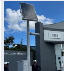
Off-grid street lighting
