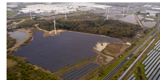
Solar power generation at the Sunderland Plant
