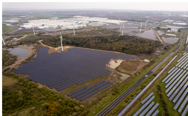
Solar power generation at the Thailand Plant
