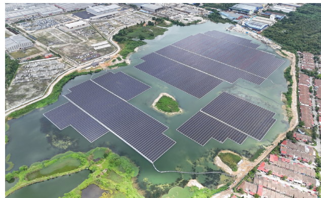
Solar power generation at the Tan Chong Motor
