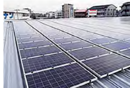
Solar panels are on the roofs of some Kanagawa Nissan dealerships. Power from the panels is supplied to dealerships through the PPS system.
