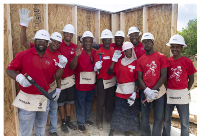
Framing a house with NNA volunteers.
