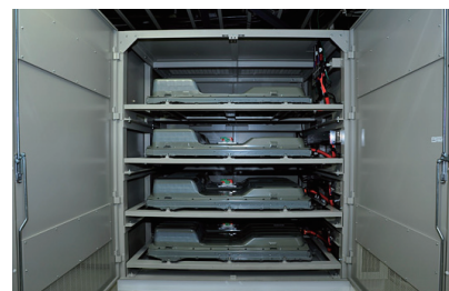
The energy storage system holds the equivalent of four Nissan LEAF batteries.
