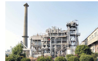
Our Oppama Plant is outfitted to recover energy from ASR.
