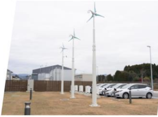
Energy management system
