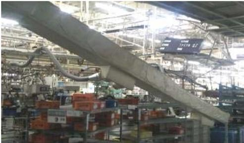
**Collapse of air ducts**
