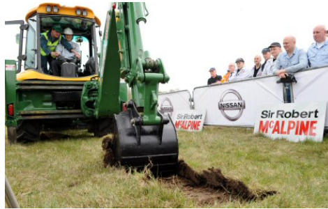
April : Ground-breaking at Sunderland battery plant, UK
