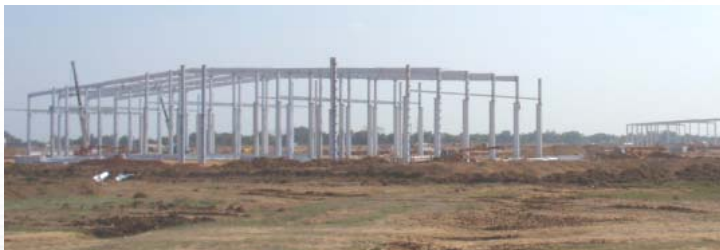
Chennai plant construction
